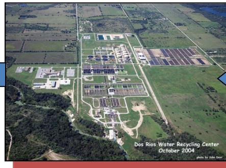
Wastewater Treatment Plant
